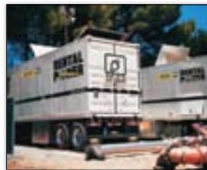
LOAD BANK SERVICE
